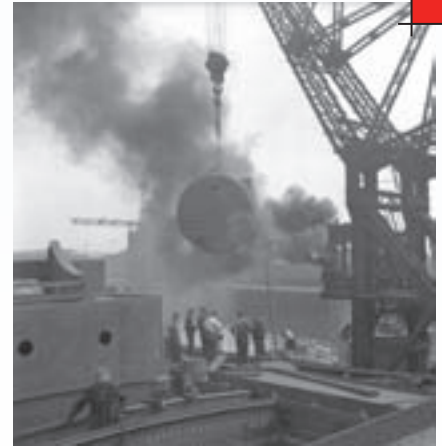
Marine crane loading boilers and engine assemblies at shipyard, 1943, Montréal, QC (photo courtesy of the National Film Board of Canada and Library and Archives Canada)
