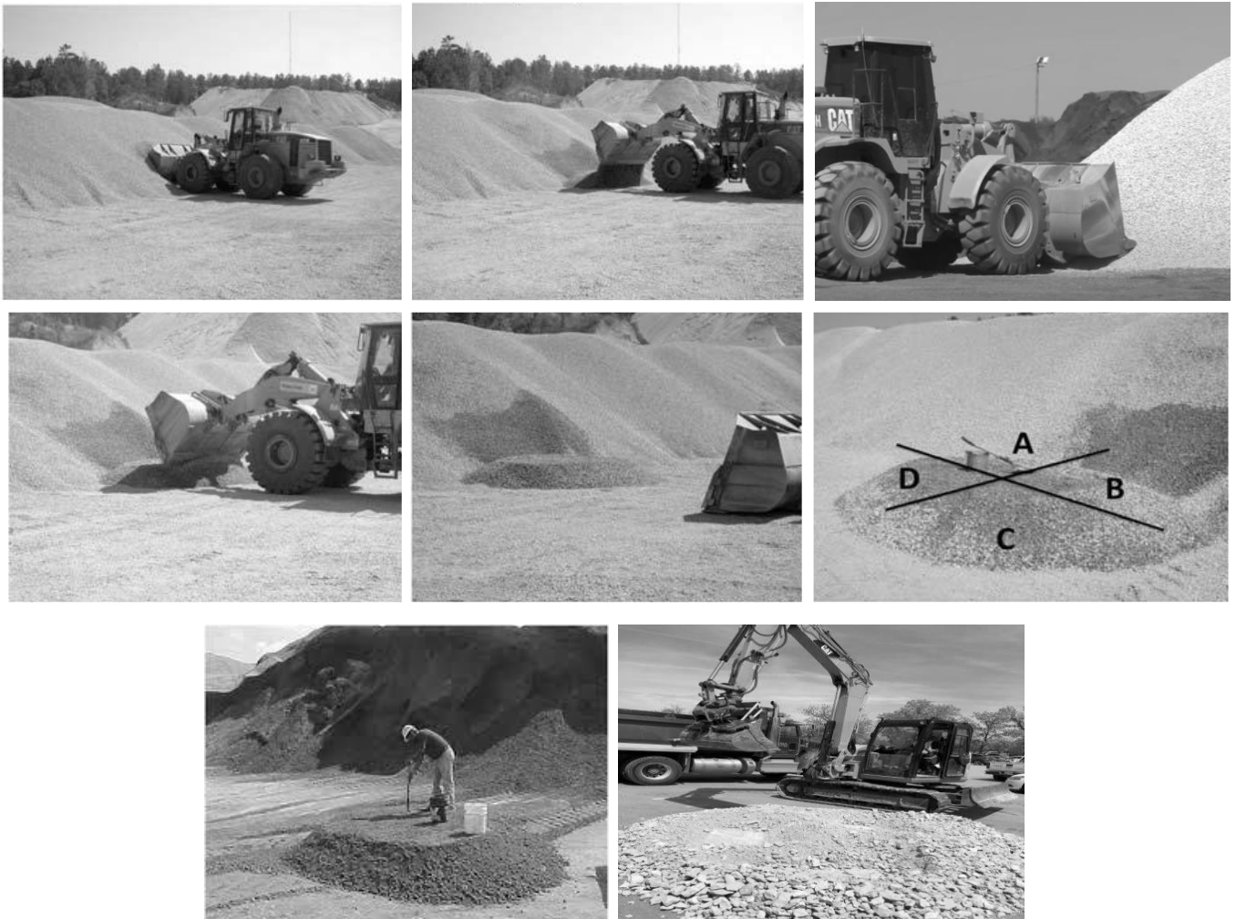
Figure 1: Sequence of constructing sampling stockpile from existing stockpile
