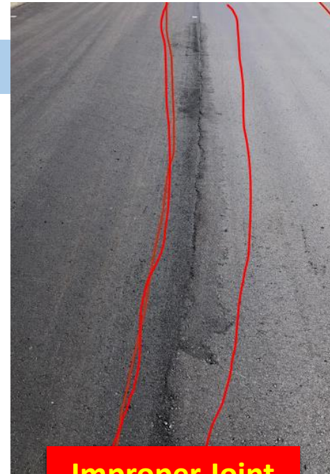
Improper Joint
