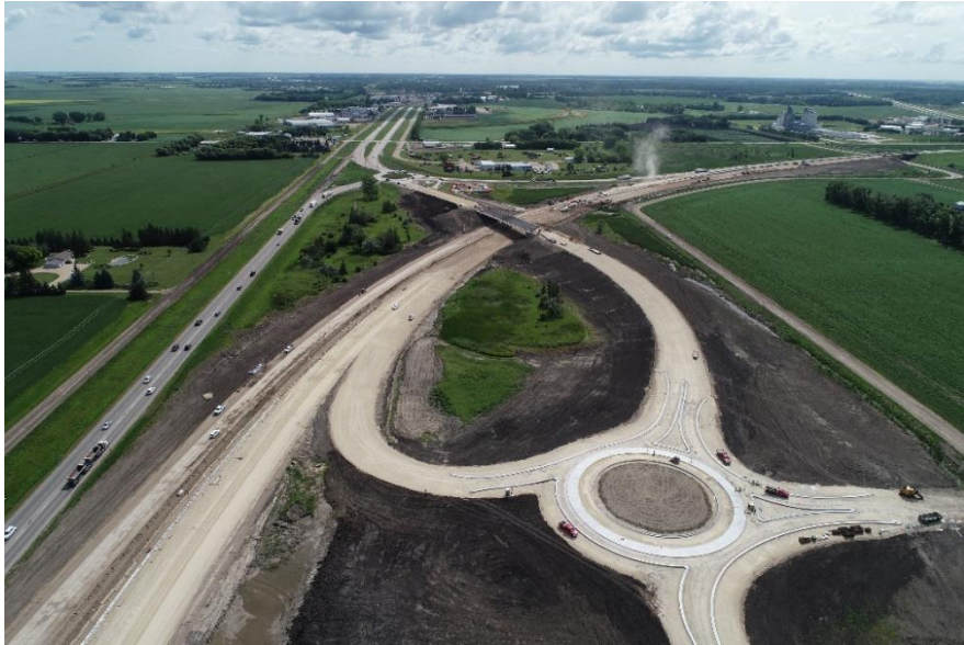
PTH 1: Portage 1A West Jct (Portage Diversion—Can Oat Road) Bituminous Reconstruction
