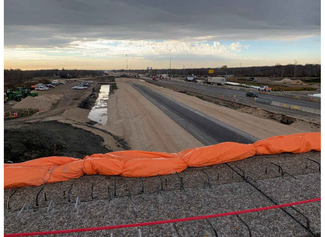
South Perimeter (PTH 100): At St. Mary's Road Interchange Construction
