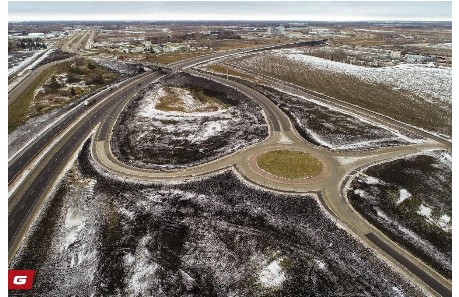
PTH 1: Portage 1A West Jct (Portage Diversion—Can Oat Road) Bituminous Reconstruction
