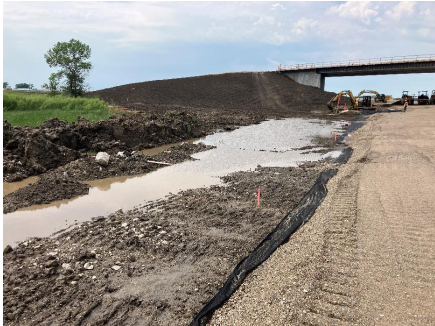
PTH 1: Portage 1A West Jct (Portage Diversion—Can Oat Road) Bituminous Reconstruction
